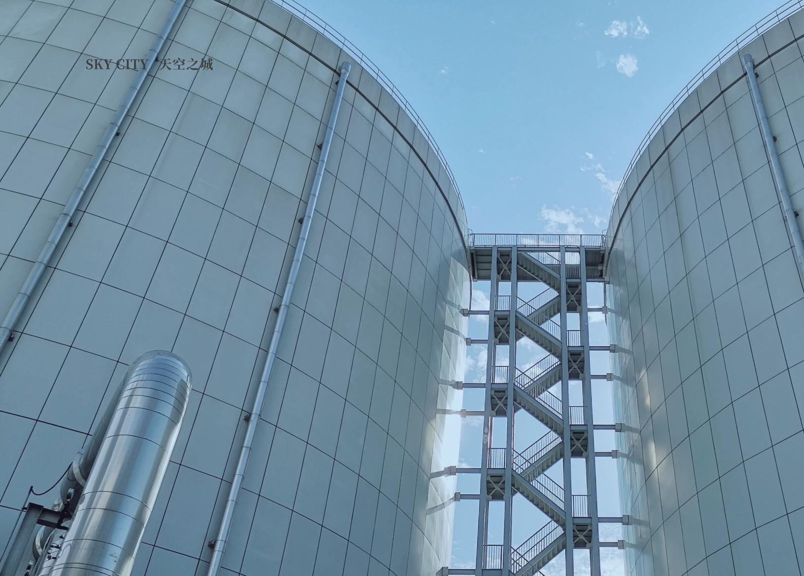
Chilled Water Storage Air Conditioning for Off-peak Power Use Helps Shanghai Pudong International Airport Reduce Peak Power Consumption by 157,000 kW·h Per Day
